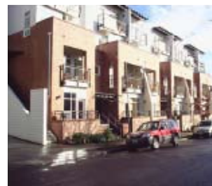
Standard 2c example. Entrances should be slightly set back from the property line and elevated two to five feet. Step backs can be incorporated to provide balcony and terrace spaces.
