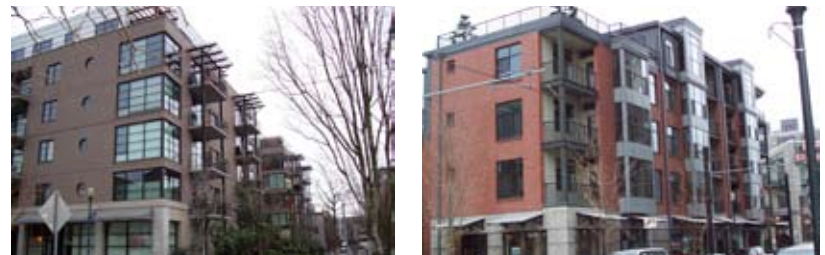
Vertical Breaks in Facade Design
