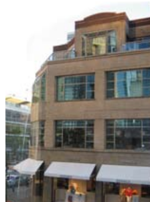
Standard 2b example. This structure is stepped back above the 3rd story providing a variation in building mass.
