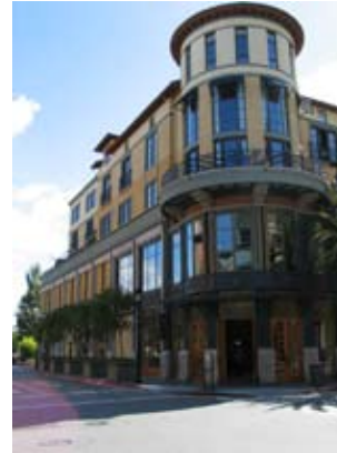
Standard 2b example. Upper levels are stepped back, providing relief from buildings
